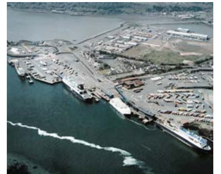
Cairnryan Ferry Terminal
